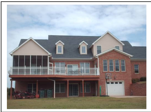
Rear of house
